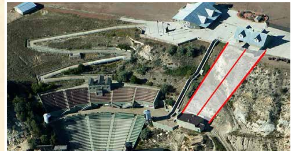
The new Incline Elevator for mobility impaired guests will be located right beside the existing escalator.
